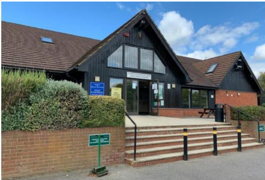
Above & Below: Photograph showing former clubhouse building
