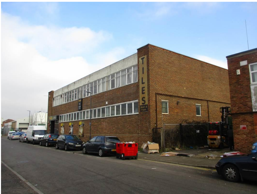
Front (west) elevation facing Brember Road
